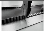
Make a cut at the edge of the lifted seam section.
