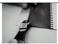
Lift the seam outwards to a right angle.
